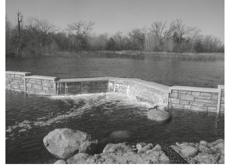
The compound weir has restored water levels and revived wildlife at Dean Lake.
